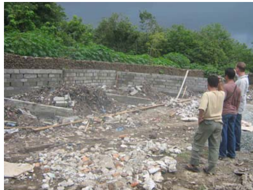
Initial construction on the composting box, Lapang final dumpsite, Aceh Barat
