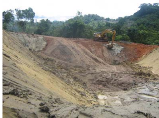
Finalization of temporary dumpsite, Gunung Tanggoh, Aceh Jaya
