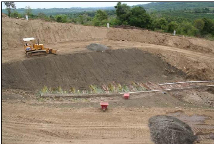
Nearing completion of engineering works for Cell 1 at Km 23 dumpsite, April 2006.
